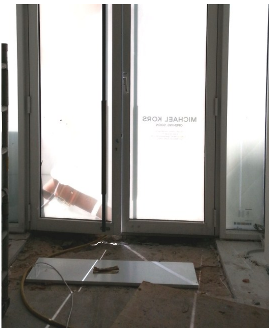
Floor Guard Antenna before pouring concrete
